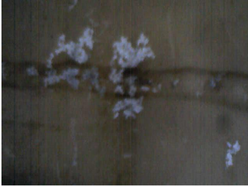
2(e) Internal Surface of Centre Weld Seam of Poor Cask: exposed aluminium
